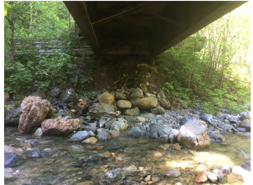
Left Bank Abutment when facing downstream
