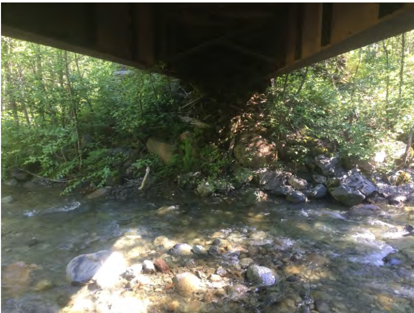
Right Bank Abutment when facing downstream
