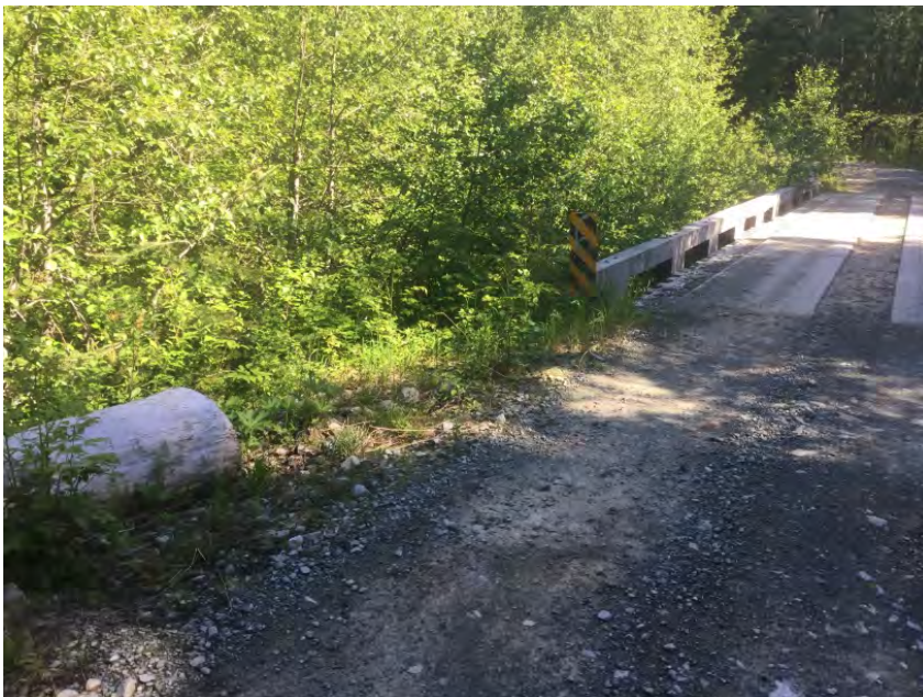
Fender log can be realigned closer to bridge
